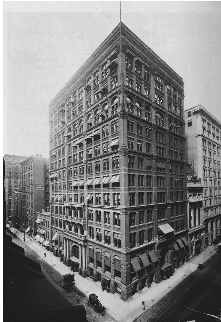
Home Insurance Building, northeast corner, 1890
